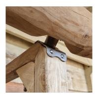
The hardware is made of stainless steel or galvanized steel to ensure durable connections with a high corrosion resistance. This robust construction guarantees long-lasting performance even in harsh environments.
